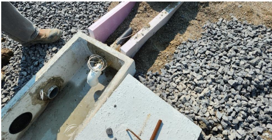
Figure 4: An example of tracer wire (white) installed around the forcemain and accessible from within the distribution box at the forcemain inlet and along a leaching bed run.
