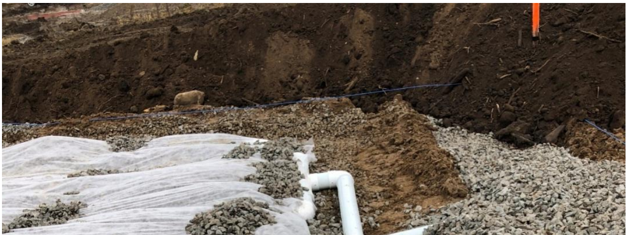
Figure 2: An example of tracer wire (blue) installed around perimeter of a leaching bed.
