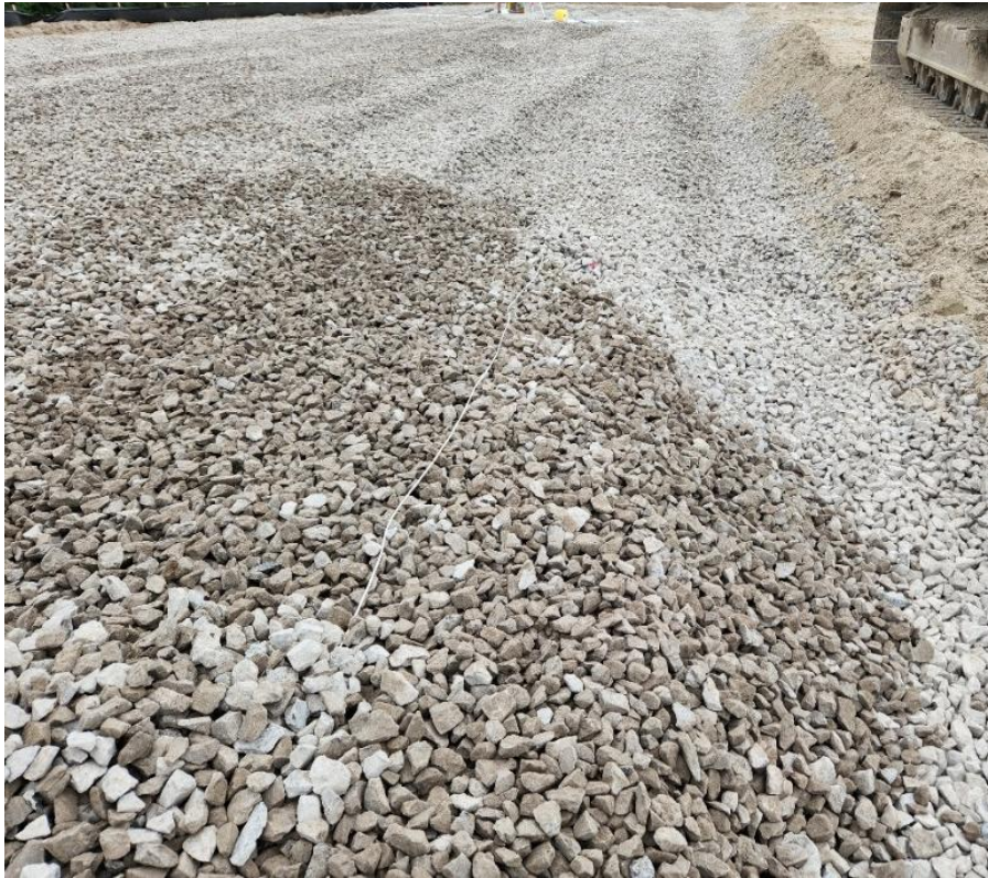
Figure 3: An example of tracer wire (white) installed around perimeter of a leaching bed.
