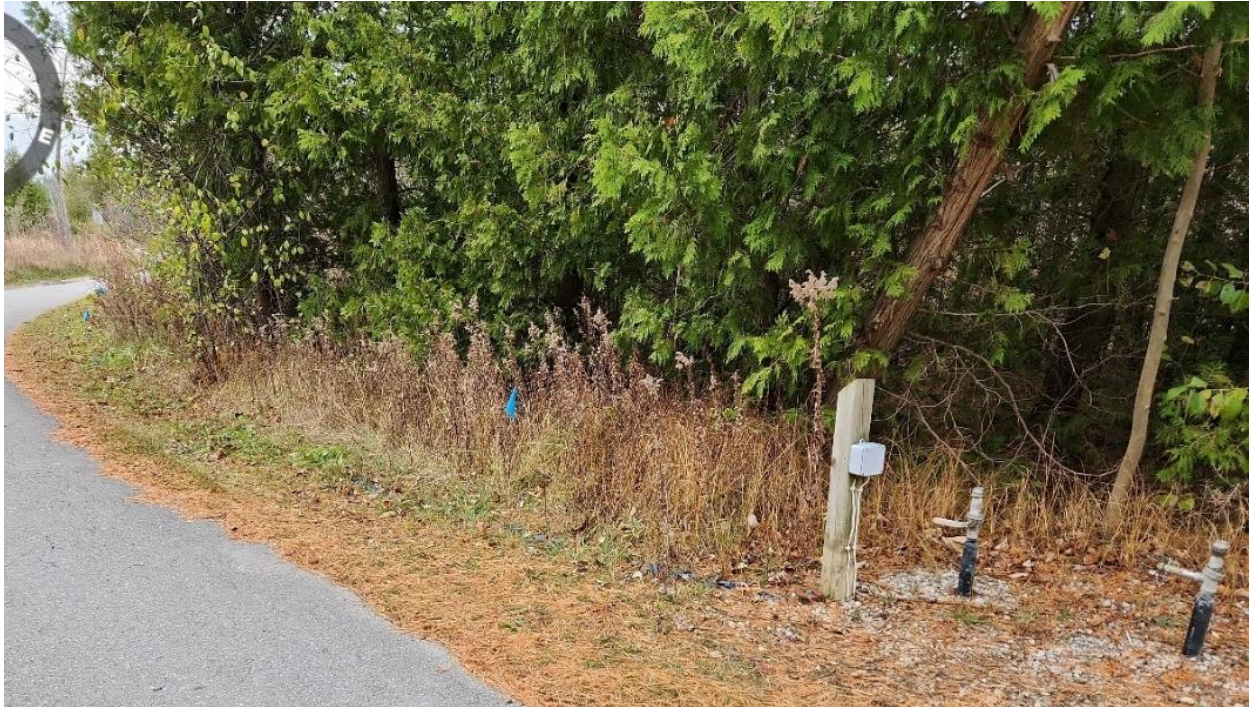
Figure 1- An example of a grey tracer box located on a wooden post.
