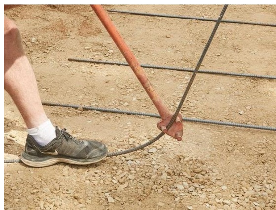
Figure 6: Rebar being bent for a corner elbow; rebar rods placed horizontally in the background.
