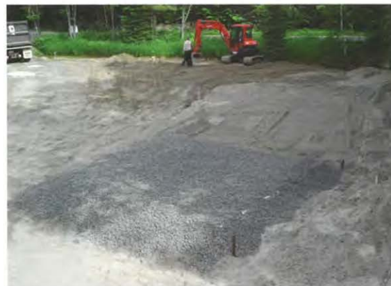
Filter bed with contact area and mantle.
