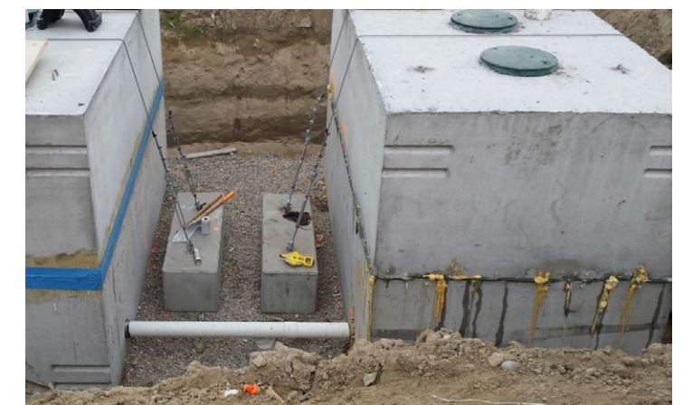
Figure 4: Anchoring Using Concrete Deadman Anchors
