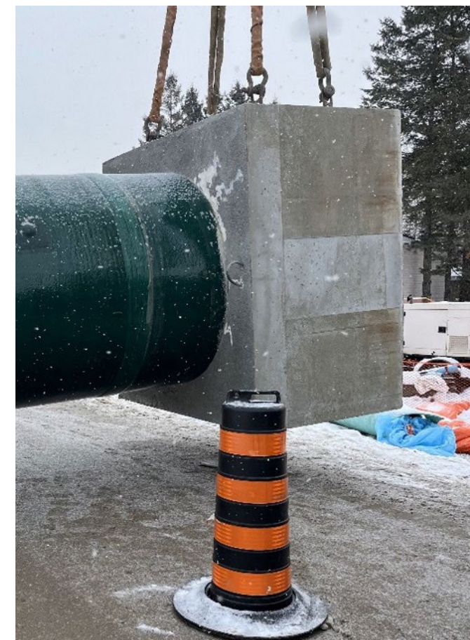
Figure 3: Prefabricated Lift Station with Concrete Ballast
