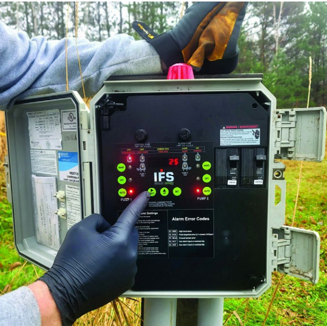
An example of a flow equalization panel from SJE Rhombus that can be helpful at monitoring and adjusting flow in vacation rental home onsite systems. (Photos courtesy of Sara Heger)
