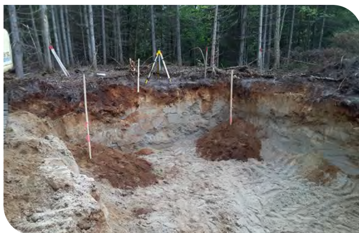
Photo 8: Bed Area Excavation with Initial B-Horizon Soil Placed
