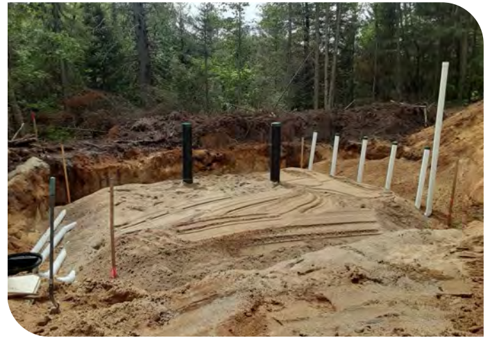
Photo 12: Final Graded System Sand Before Covering With Backfill
