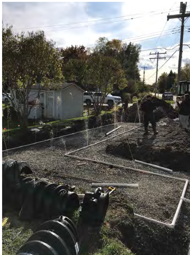
FIGURE 1: SBT INSTALLED DOWNSTREAM FROM AN ECOFLO STB-650BRA
