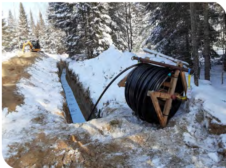
Photo 5: Pipe Roll for Laying Pipe
