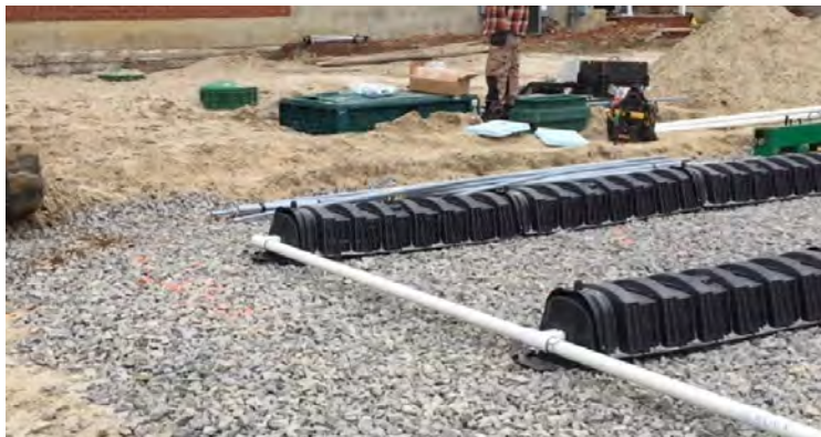
FIGURE 2: ECOFLO STB-840BRA INSTALLED WITH AN SBT
