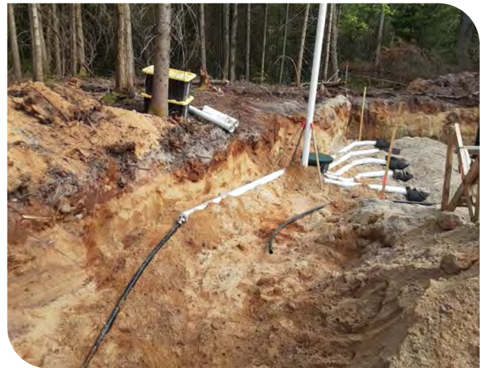
Photo 13: Pressure Pipe Connection to D-Box and Distribution to Bed
