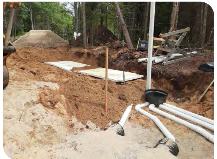
Photo 14: Backfill and Insulation Over Pipe at D-Box Prior to Final Cover
