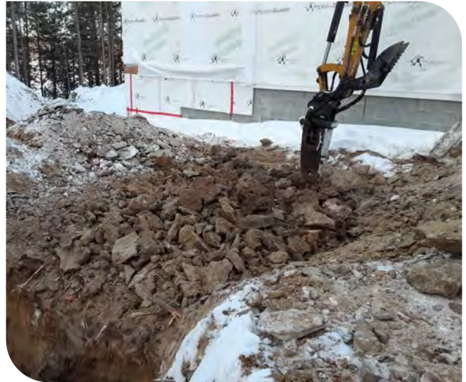
Photo 2: Frost Breaking for House to Tank Connection
