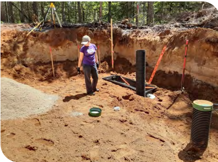
Photo 10: Sample Device for Enviroseptic Bed and Start of System Sand Fill
