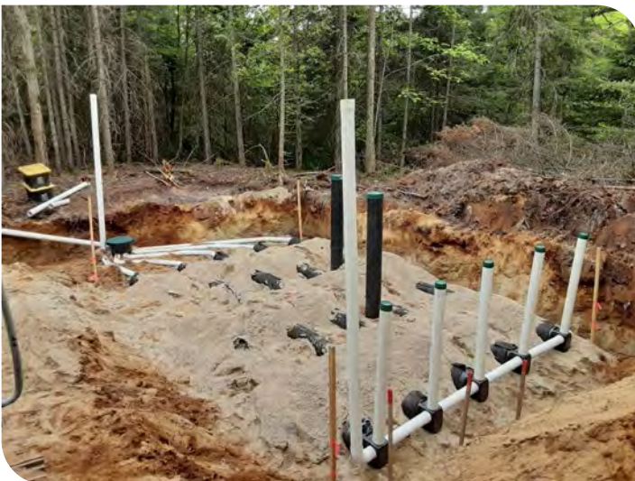
Photo 11: Enviroseptic Bed with Pipe, Connections to D-Box and Sample Tubes and Vents
