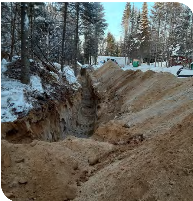
Photo 3: Initial Pipe Trench Excavation
