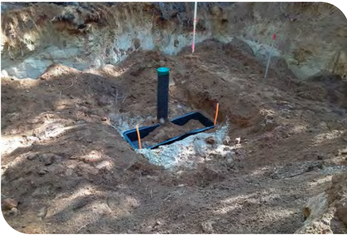
Photo 9: Sample Device Under B-Horizon Soil Layer
