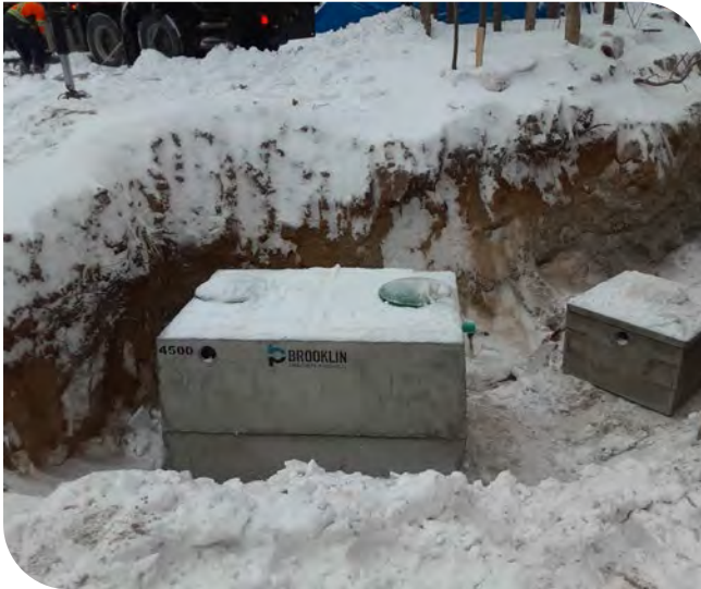
Photo 1: Tank and Pump Chamber Placement
