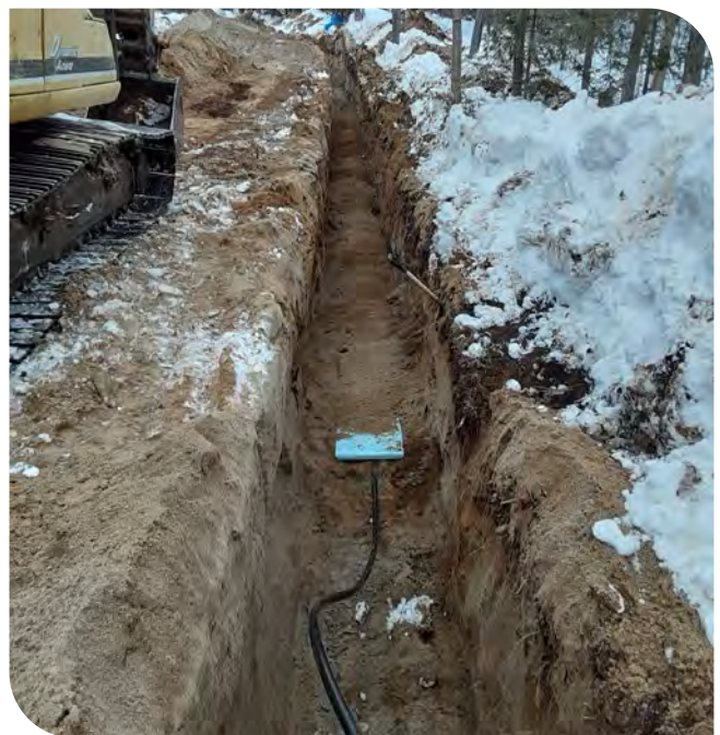
Photo 4: Laying Pipe and Insulation
