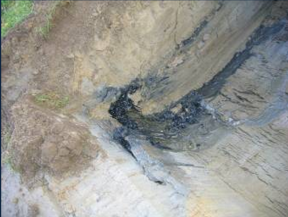
Effluent breaking through during mantle install
