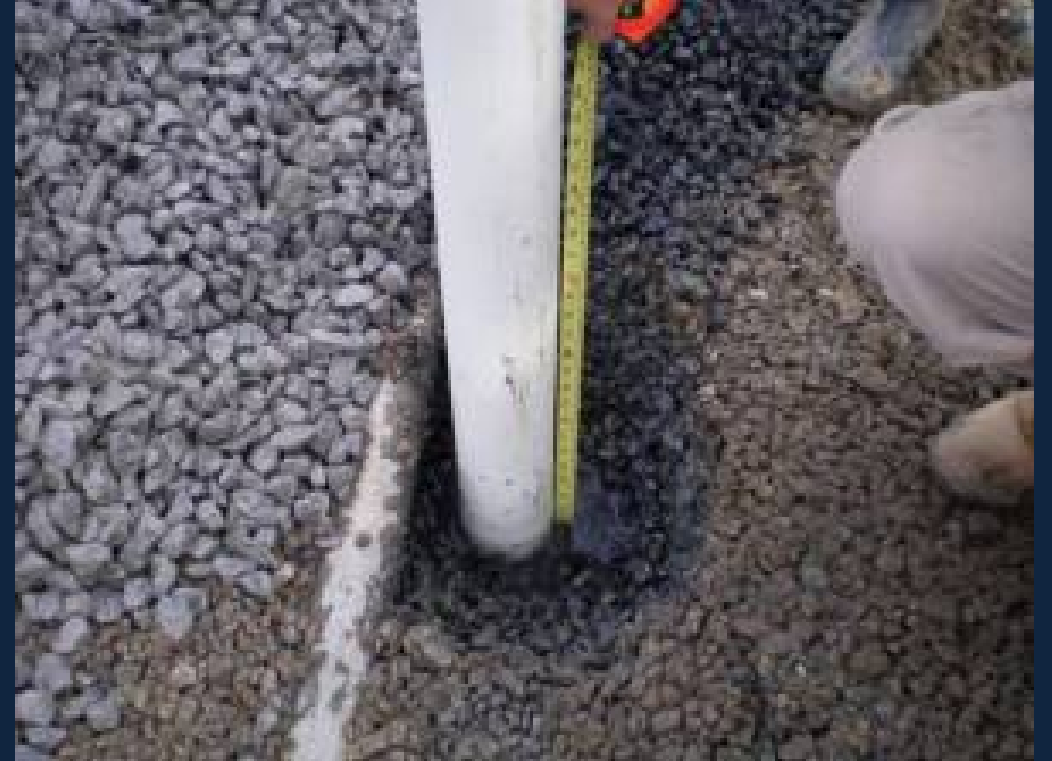
Peizometer installation
