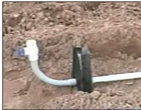
Figure 2: Sweep 90 with ball valve and end cap
