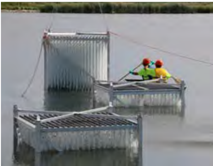
BioCord reactors are installed directly into the treatment lagoon, helping to reduce capital costs and operator oversight.
