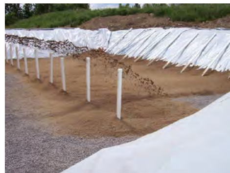
Rene Goulet's reed beds was built first by installing cement sand over the two types of gravel, with a felt liner at the bottom to ensure the bed would not contaminate the water table.
