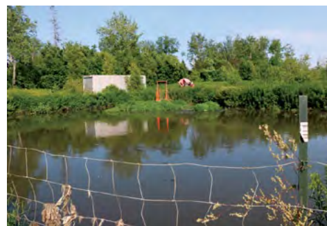
This tiny lagoon is the first stop for septage at Baird Septic Tank Pumping's treatment facility in Nova Scotia. Floating sludge, as seen in the middle, will be skimmed off. Water from this lagoon passes through a filter and drains to a much larger lagoon.
