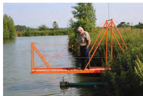
Allan Baird looks down from a wharf overlooking his largest lagoon. The green pipe leads towards a filter that traps solids and drains to a third, smaller lagoon, which, in turn, drains into a wetland.
