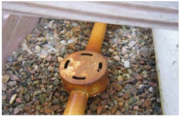
Iron staining on a lateral system.
