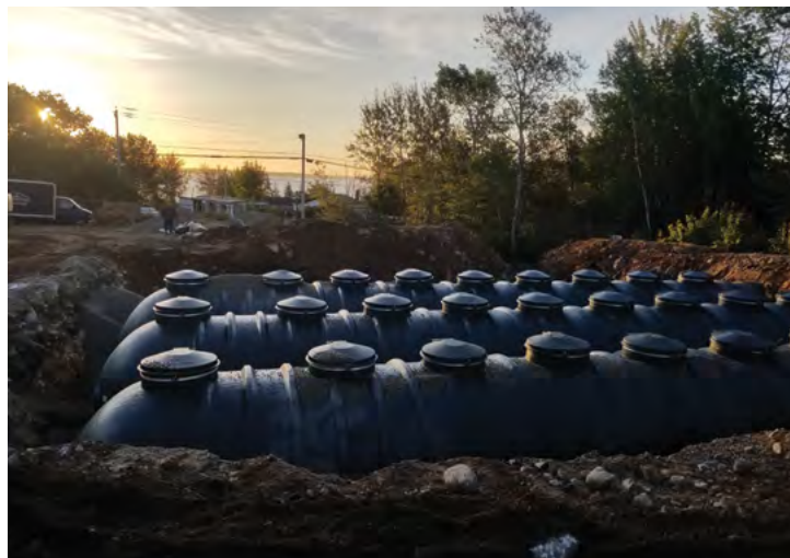
Fibreglass Treatment Tank Excavation
