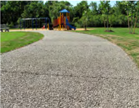
Permeable pavement used on a park pathway (City of Hamilton)
