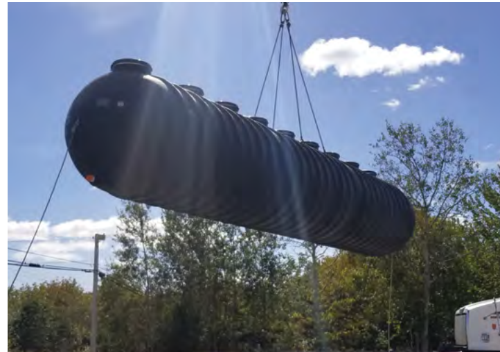
Waterloo Biofilter Fibreglass Treatment Tank Placement
