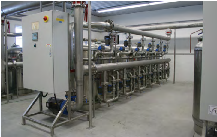
Figure 4: Filtration trains at the drinking water treatment plant for JW Marriott Resort.
