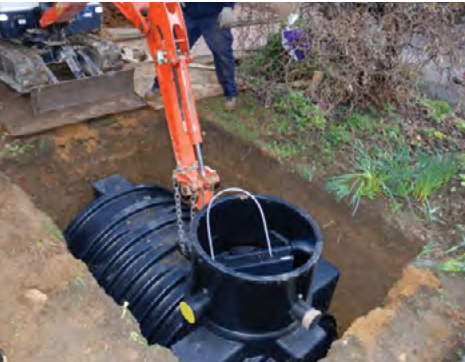
Look familiar? A water storage tank install. ( houseplanninghelp.com )
