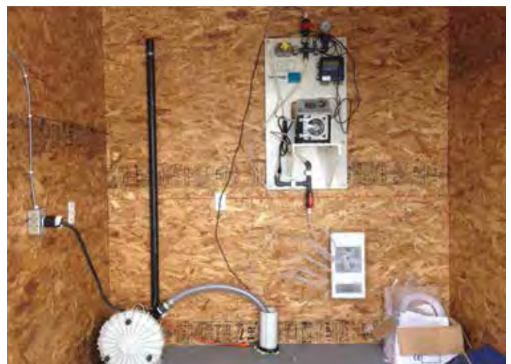
PH ADJUSTMENT SYSTEM AND BLOWER
