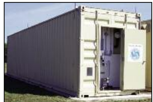
Figure 2. WATERLOO BIOFILTER SC-40 configuration that can treat 25 three-bedroom houses or the equivalent. Two SC-40s are used at Truck Stop A.
